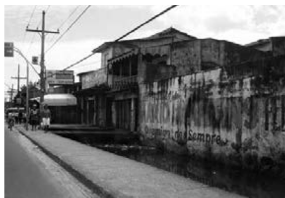
Photo 30 Guamá (3): Sanitary conditions
